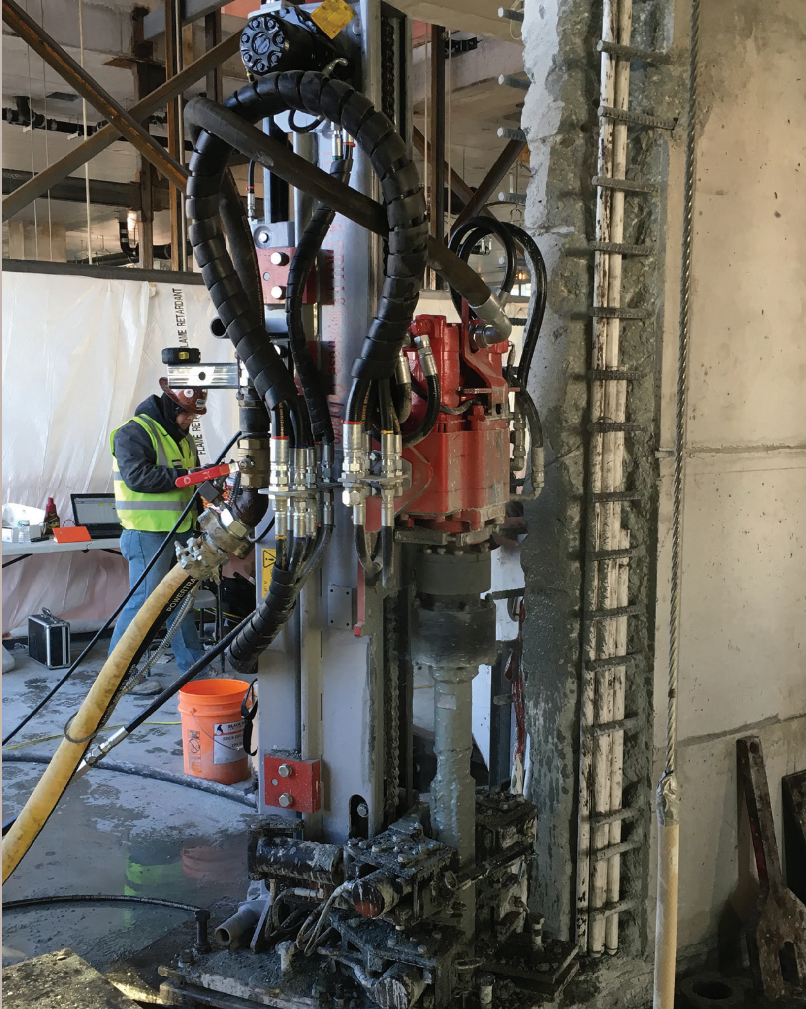
PD550 PORTABLE DRILL INSTALLING MICROPILES IN A HIGH RISE, BETWEEN FLOORS.
